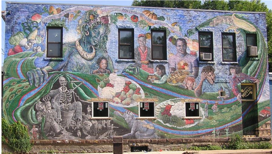
Existing mural running parallel to Mifflin Street
